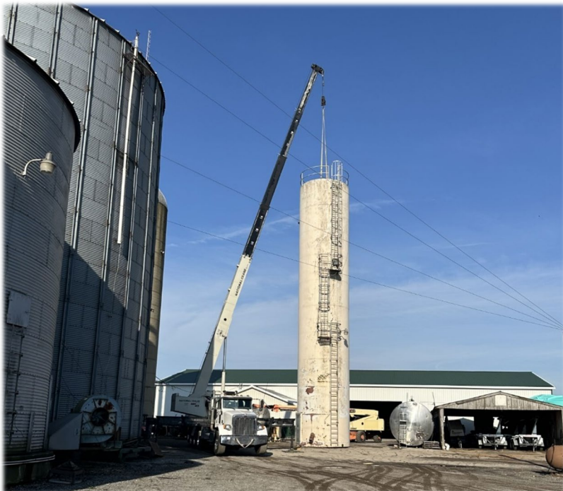
Above the Crain is moving the metal silo. This is being moved behind the seed plant where the new bins were just assembled.
