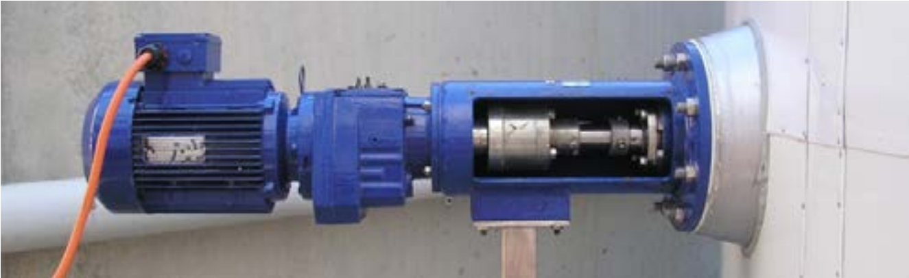
Figure 4. Example of a side-mount horizontal motor for mixing (Source: J. Lechman, J&R Consultants, Ltd., Winnipeg, MB, Canada).
