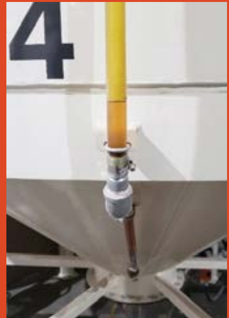
Figure 5. Example of external measure of existing tank volume (Source: J. Lechman, J&R Consultants, Ltd., Winnipeg, MB, Canada).
