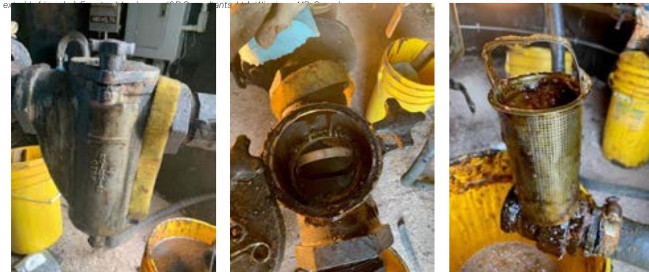
**Figure 11.** Example of sediment collected from an oil storage tank. (Source: J. Lochman, I&P Consultants)
